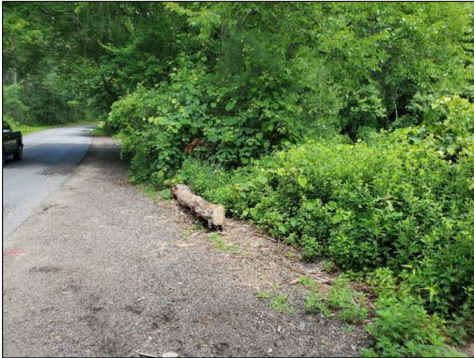
Photo No. 11. Crest and upstream shoulder from STA 2+45 looking right. Note the gravel upstream shoulder used as a parking area.
