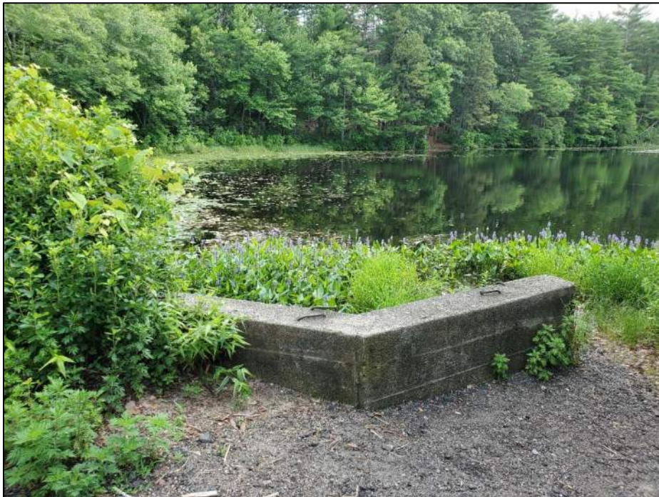
Photo No. 30. Overview of the impoundment from the historic LLO inlet.
