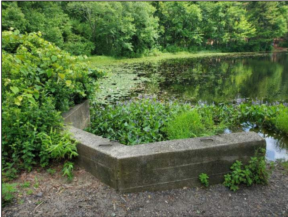
Photo No. 25. Historic LLO intake structure. Note the vegetation growing in the area of the historic intake.
