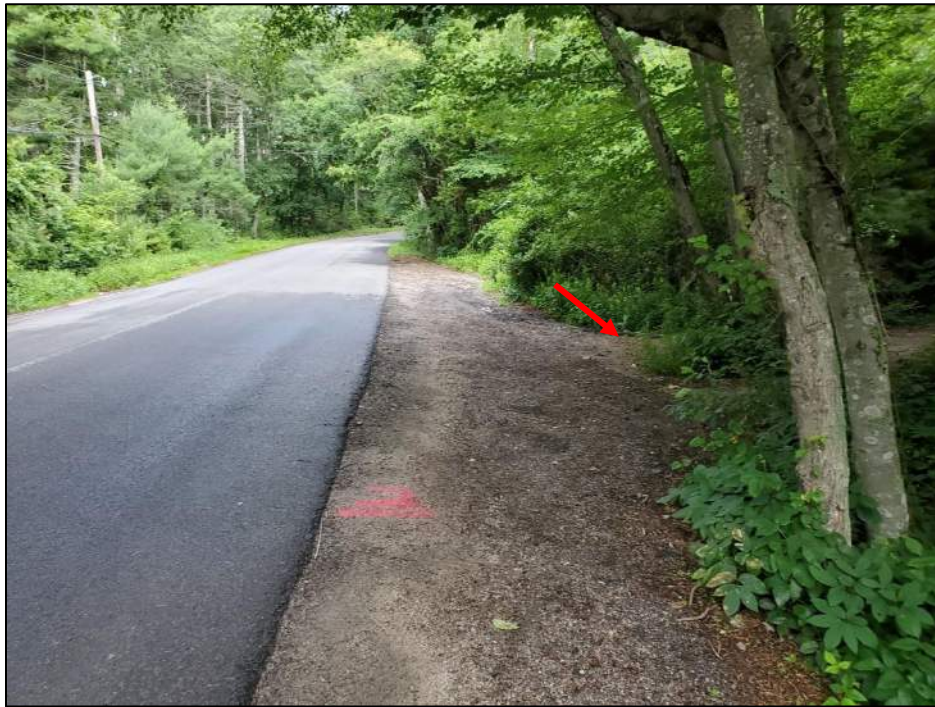
Photo No. 12. Upstream crest contact with right abutment. Note the upstream footpath roughly marking STA 3+20 (arrow) and the right abutment.
