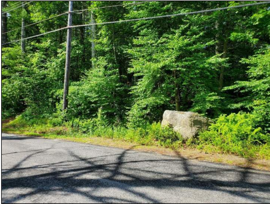
Photo No. 9. Downstream crest contact with the left abutment. Note the large boulder roughly marking STA 1+00.
