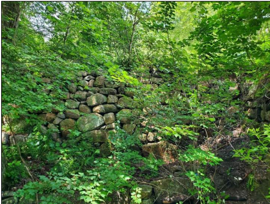
Photo No. 20. Downstream slope at STA 3+00 looking right. Note the dry set stone masonry wall.
