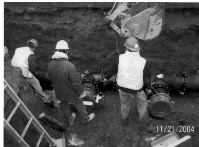
Tiverton Fire District Interconnection at Fall River
