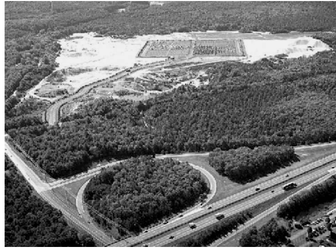
AMGEN'S temporary parking lot built over gravel pit in BRMA
