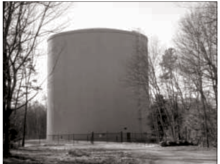
Kent County Water Authority's 3-million gallon tank in the Big River Management Area
