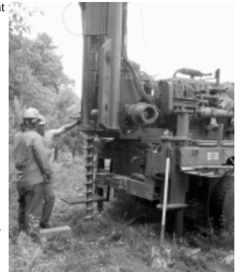
Groundwater well drilling
