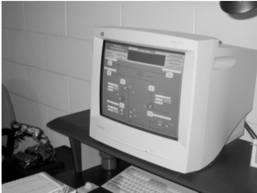
Scada - United Water RI
