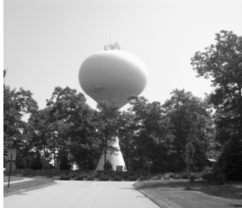
Kingston Water District Tank
