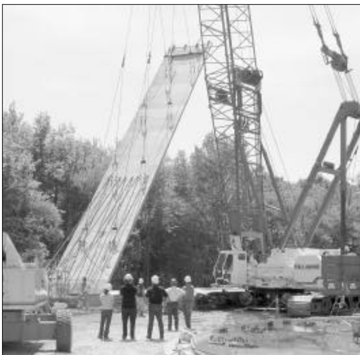
Water storage tank construction in the Big River Management Area
