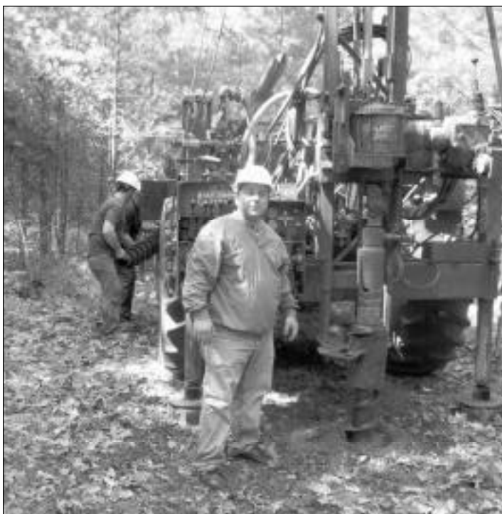
Board staff overseeing well testing
