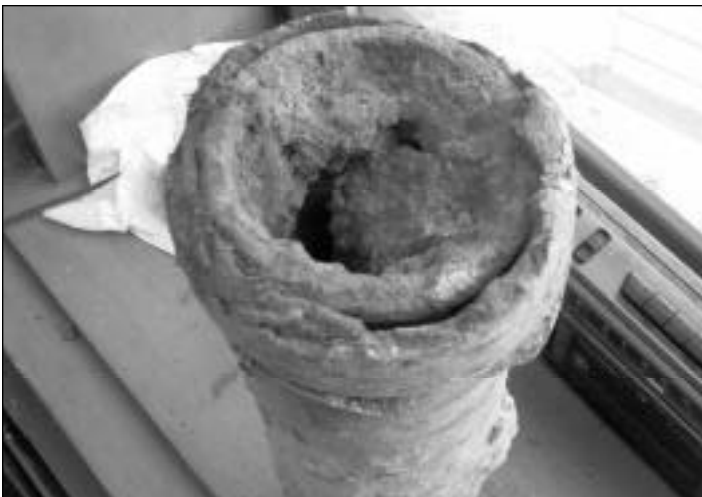
Iron-corroded water main clogged with sediment
